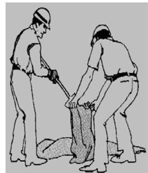
The shoveler should carefully release the rounded shovel full of soil into the throat of the bag. Haste in this operation can result in undue spillage and added work. The use of safety goggles and gloves is desirable and sometimes necessary.
